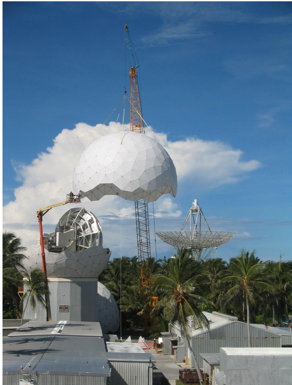
**Figure 8.** The Millimeter-Wave Radar (MMW) antenna is seen in the foreground as a new GoreTex® radome was installed in 2003.
