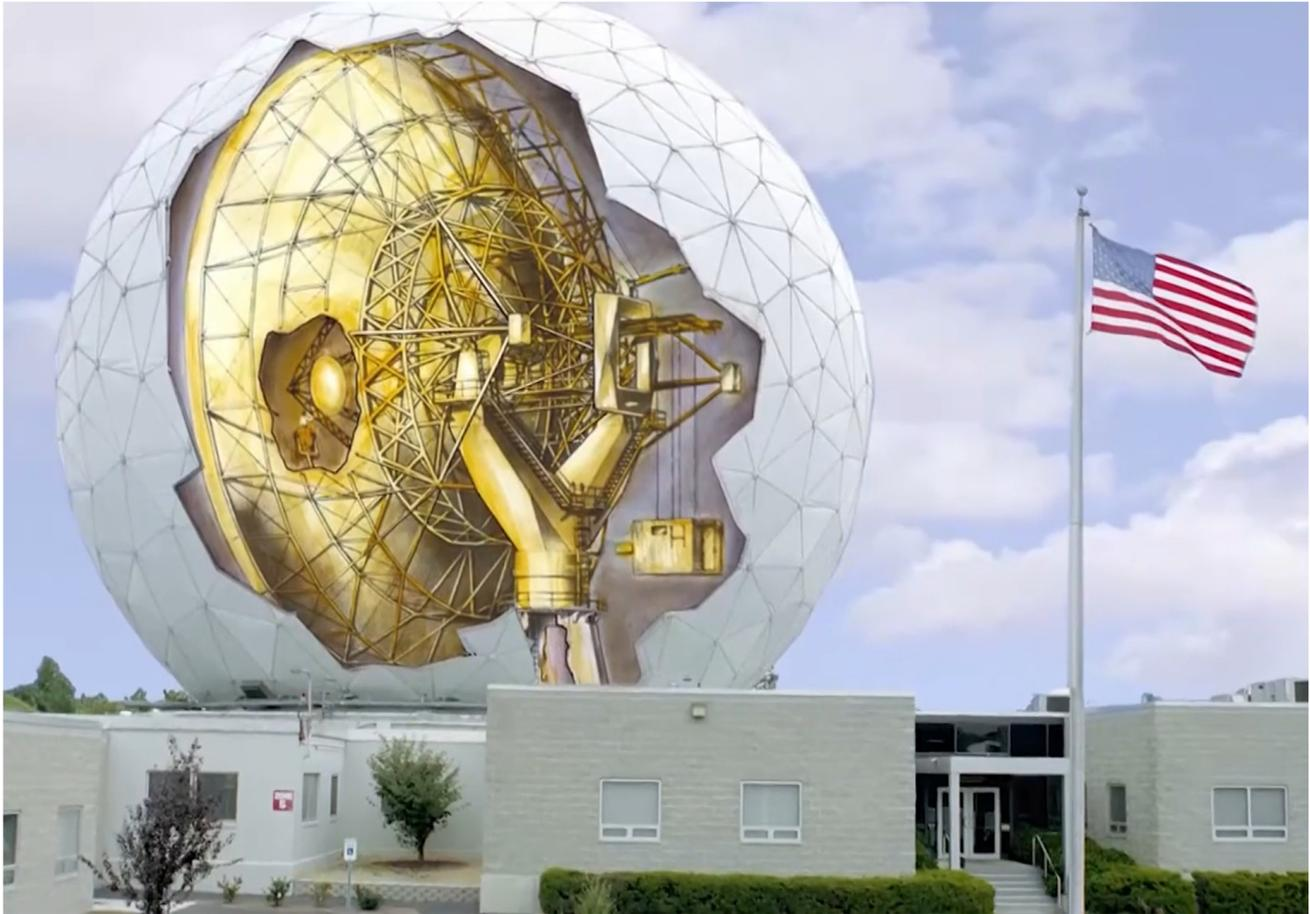
**Figure 3.** The Haystack antenna as it stood from 1964 to 2014 in a cut-away view. The figures pictured near the subreflector provide a human scale. An RF box can be seen being hoisted into place for insertion at the antenna feed.
