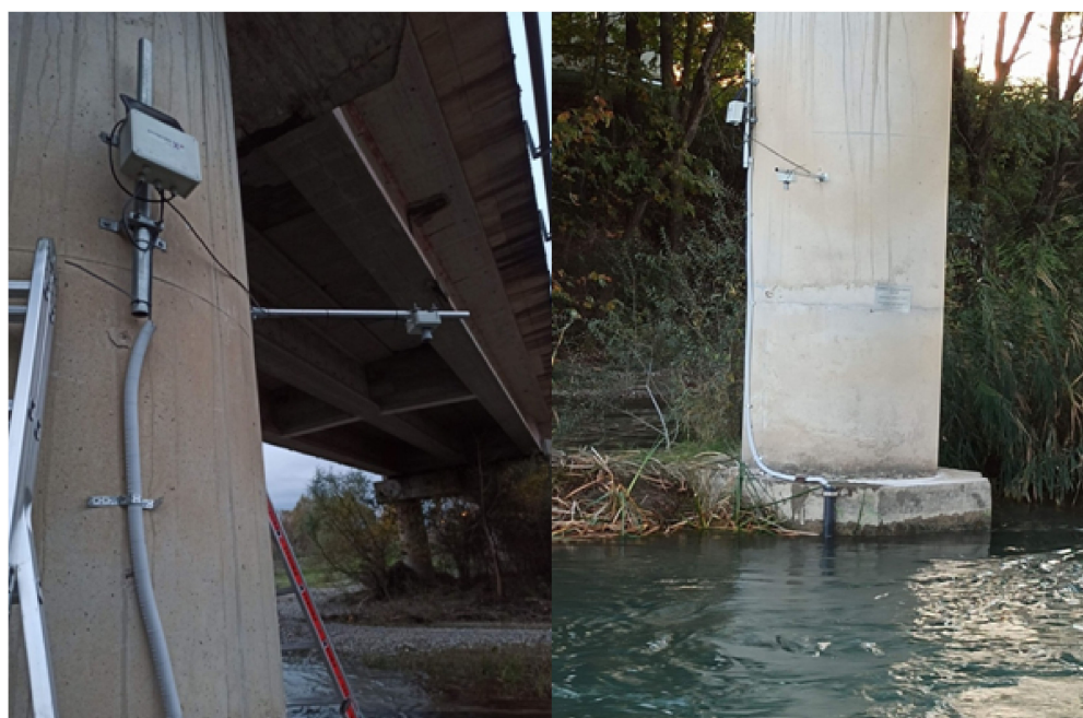
Figure 1. A typical installation of an Hellenic Centre for Marine Research (HCMR) automatic station for water monitoring: the solar panel on the pier column (left) and the instrument with the sensors in the pier's bottom (right).
