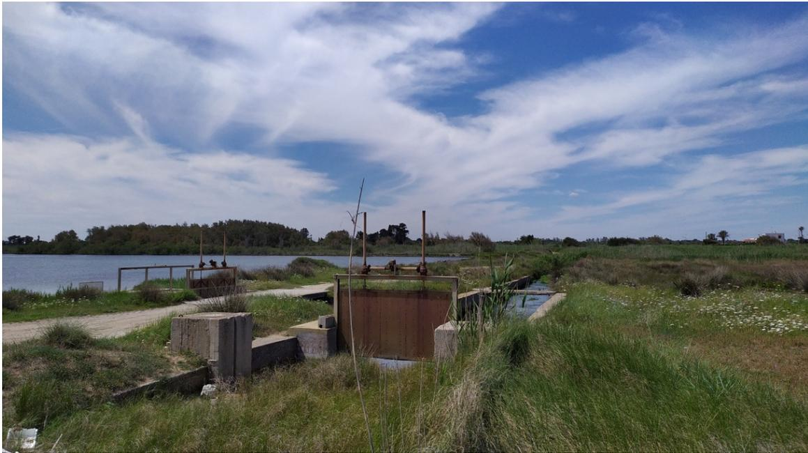
**Figure 4.** The water of Giammatteo Channel is canalized into the sea or in the Acquatina di Frigole lagoon through closed system of dams.
