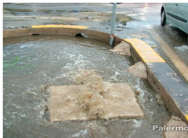
**Figure 7.** Manhole overflow at Piazza Castelforte. Source: web ([www.palermotoday.it](http://www.palermotoday.it) accessed on 27 October 2021).
