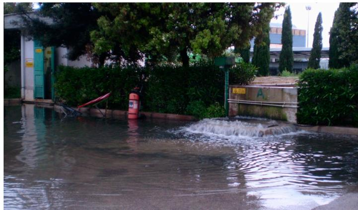
Figure 9. Overflow of the reception tank at the Water Treatment Plant.
