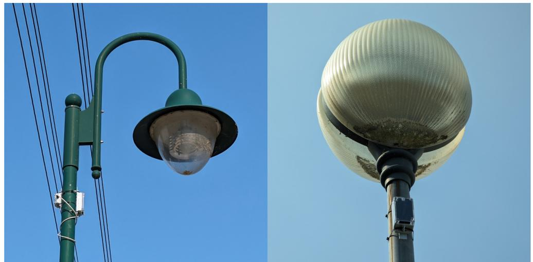
**Figure 11.** Two types of lamps in the deployment, outfitted with our sensors. These are also exemplary for two major types of designs: light source centered on the pole and offset via a boom fixture.
