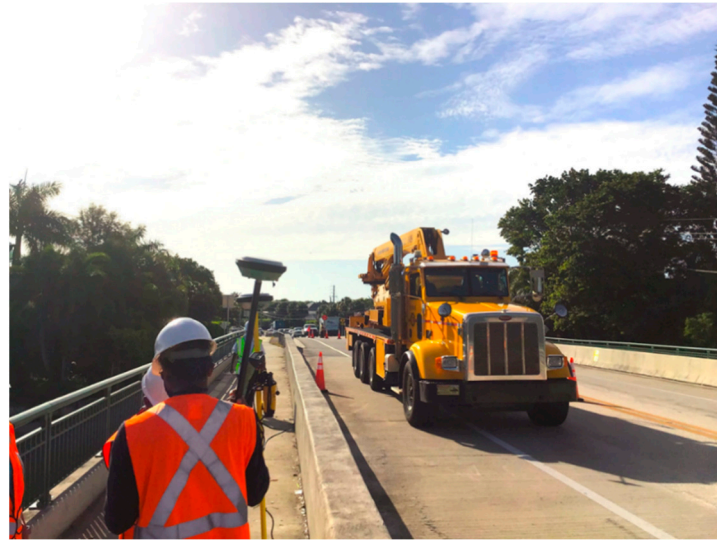
Figure 13. Snooper truck used for underwater scanning of highway bridge—Little Lake Worth Bridge, Florida.
