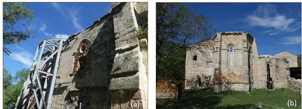
**Figure 2.** Views of the monastery of Santa María de Bonaval from the south (a) and the east (b). The building shows a marked anisotropy of decay: the south and west sections of the building show more overall structural failure. The south and east sections show the largest proportion of salt-related decay forms. Nevertheless, the east part of the building is the best-preserved area.
