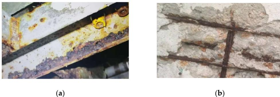
**Figure 1.** Corrosion in structural and reinforcing steels. (a) structural steel; (b) reinforcing steel.
