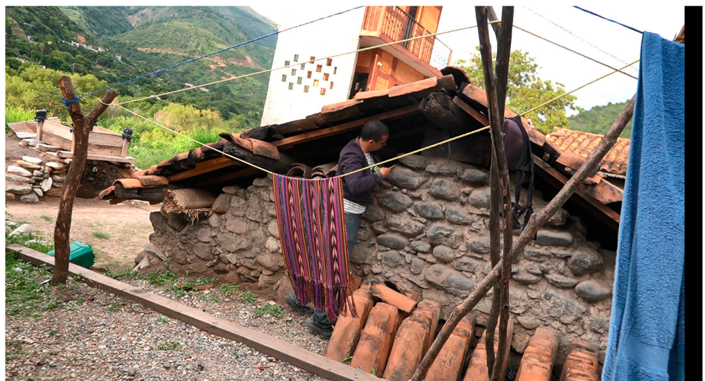
Figure 22. MSS-2 salt kitchen; the wall made from stucco and stones can be seen. It shows a rudimentary construction process without any internal structure. Author (2022).
