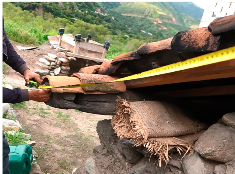
Figure 24. Salt kitchen extended roof structure, covered by Spanish tiles. The wear can be seen due to the black spots from both moisture and constant cooking inside the kitchen. Author (2022).
