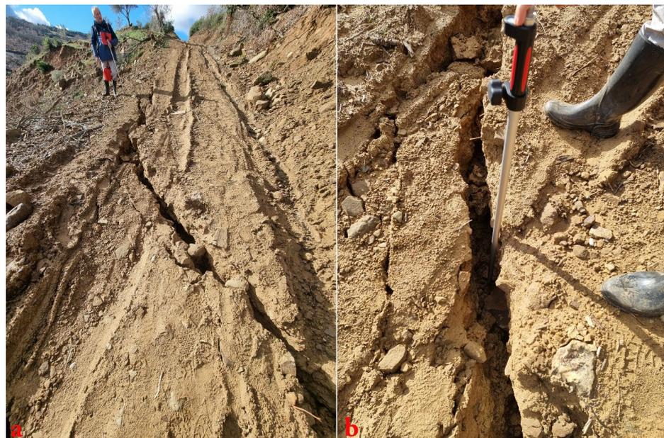
**Figure 14.** Field observations. (a) Spatial distribution of the crack across the road (b). In-depth erosion along the crack.
