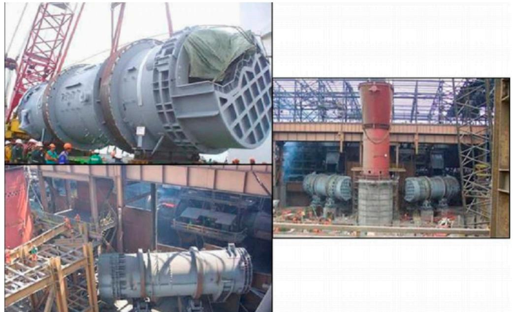
**Figure 5.** Rotary holding furnaces installation at Ilo Copper Smelter in Peru [12] (reprinted with permission).
