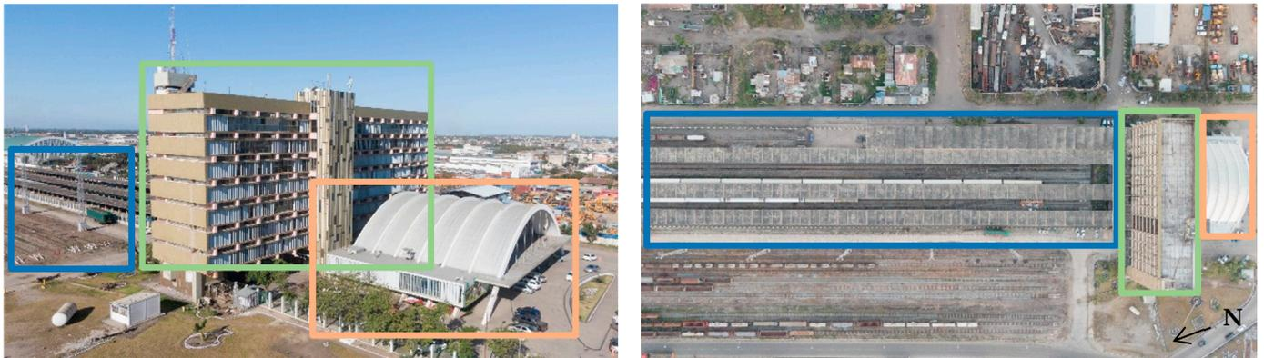
**Figure 3.** Aerial photos of the station: atrium body in orange, administration body in green, and platforms zone in blue.
