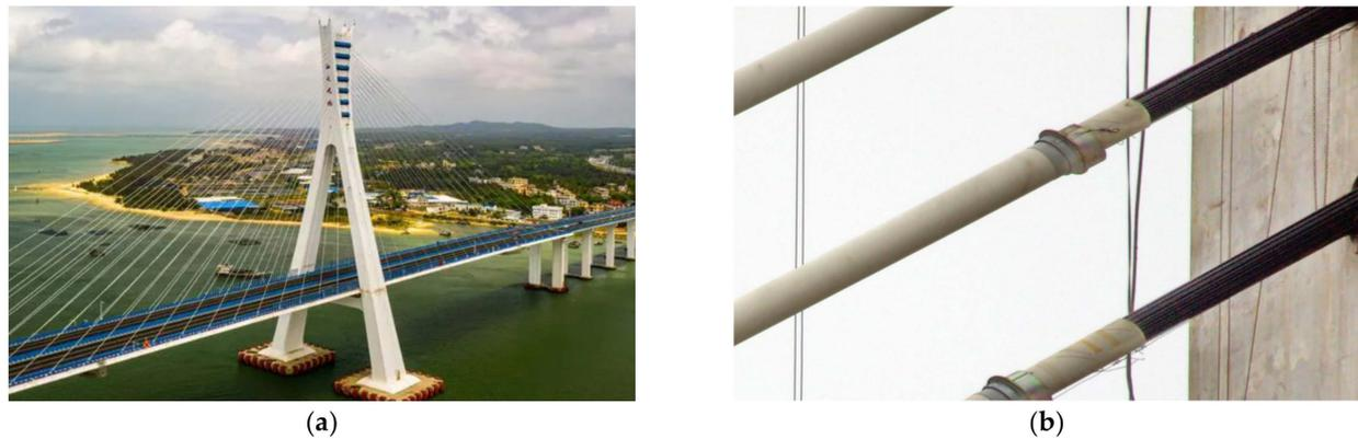
**Figure 2.** Schematic diagram of cable-stayed bridge. (a) Aerial photograph of the main bridge of a cable-stayed bridge; (b) the schematic diagram of the stay-cable sheathing and steel wires.
