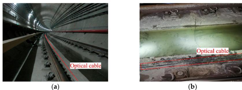
**Figure 2.** Optical cable installed on the surface of track beds: (a) a global perspective and (b) a zoom-in view.
