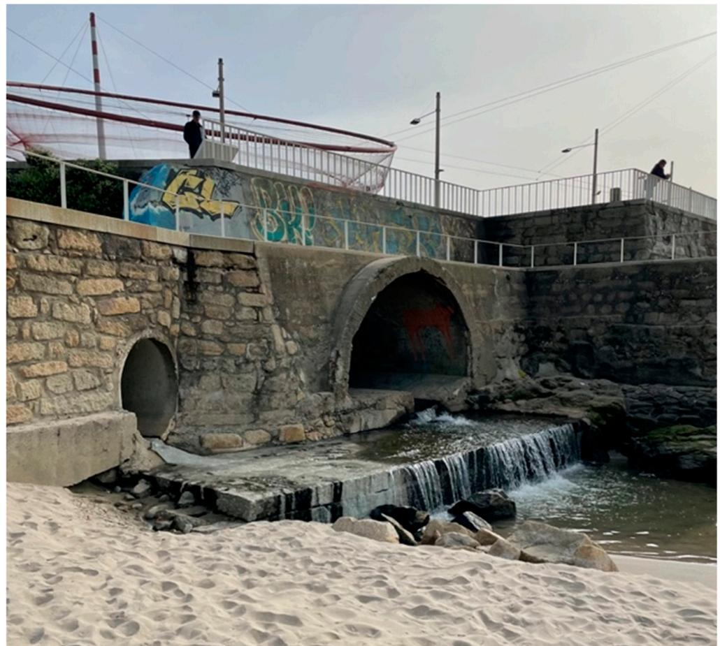
**Scheme 1.** Tunnel on the right: final section of Riguinha stream, concrete pipe 4.4 m wide and 2.3 m high. On the left: smaller concrete pipe corresponding to the water drainage of Brito Capelo Street, Matosinhos.
