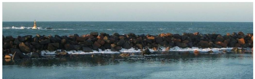
Figure 9. Wave transmission flow along core/armour interface (the author, January 2008).
