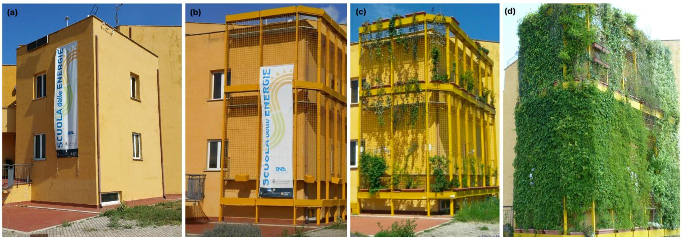
**Figure 1.** Consecutive steps in the installation of the green wall at the ENEA “green” building demonstration platform. (a) The building without the vertical green wall installation; (b) yellow stainless-steel infrastructure with three series of planter holders, respectively at the base and on the 1st and 2nd floor of the building; (c) transplanted plants attaching themselves to the lattice infrastructure (April 2017); (d) plants completely covering the infrastructure (June 2019).
