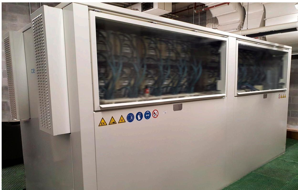
**Figure 1.** A containerised VFB system.
