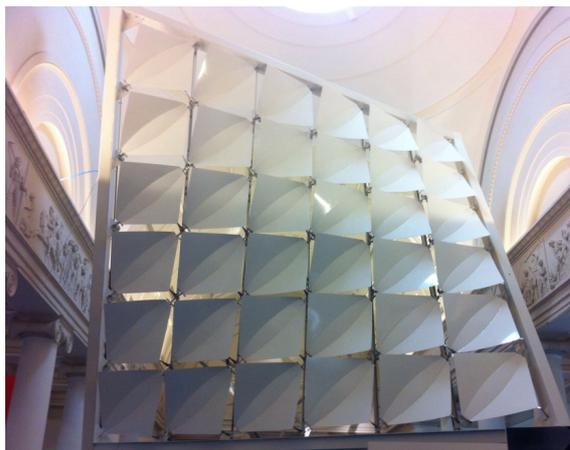
**Figure 22.** The demonstrator shows an application of Flectofold as a shading device. It consists of 36 Flectofold elements in an open state, each measuring 1 m × 1 m.
