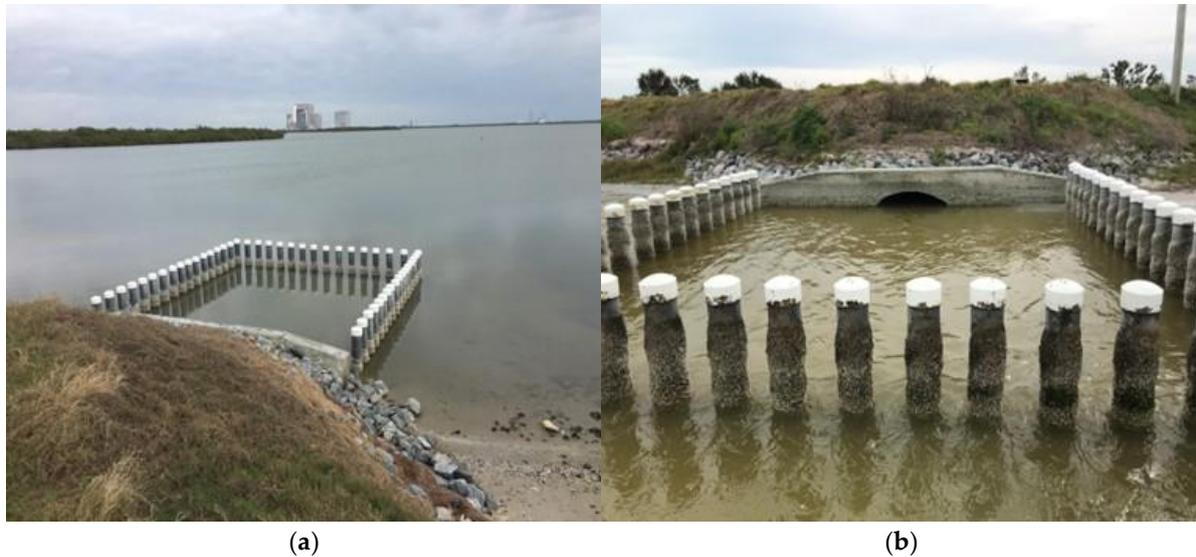
**Figure 2.** Integrate-Transfer-Launch Impoundment culverts (a) Manatee exclusion bollards installed around the ITL impoundment culverts.; (b) ITL culvert surrounded by bollards which have been fouled by barnacles near the water line.
