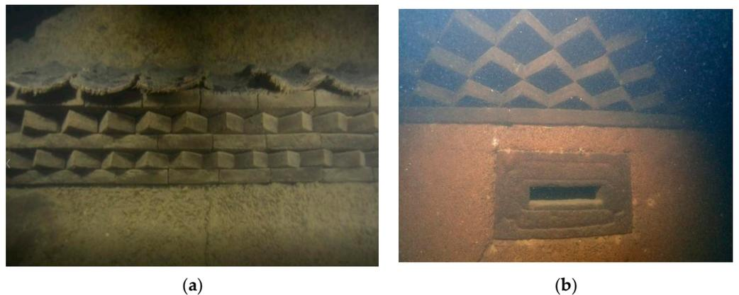
**Figure 55.** (a) The gray sand wall of a sijaolou building. (b) Defensive gun-holes on the wall of a sijaolou building.
