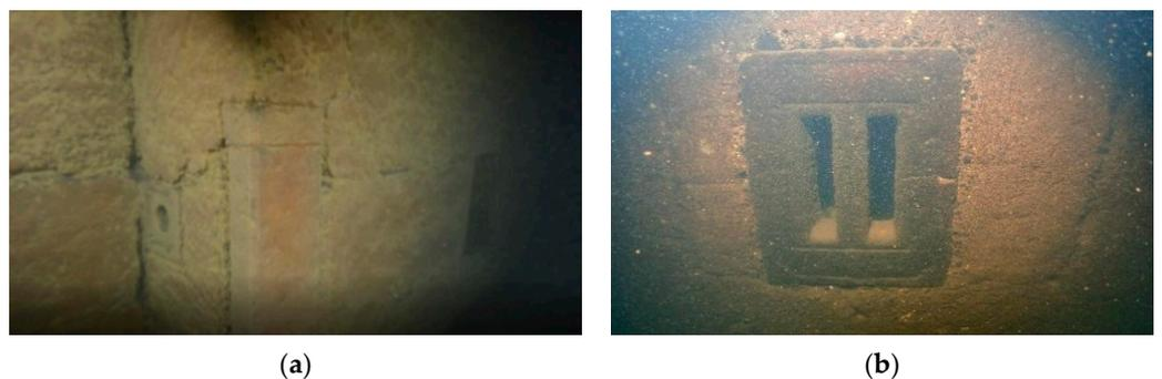
**Figure 56.** The solid wall structure of a sijaolou building constructed with rammed gray sand. (a) on the corner of the wall. (b) in the middle of the wall.
