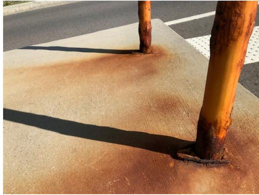
**Figure 10.** Example of watery-looking rust stains that resulted from oxidation of water-soluble ferrous chlorides formed in deep defects and cracking in the protective coating.
