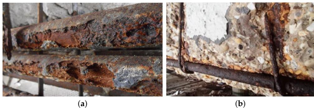
**Figure 2.** Deterioration of RC sections due to (a) chloride-induced and (b) carbonation-induced corrosion of reinforcement.
