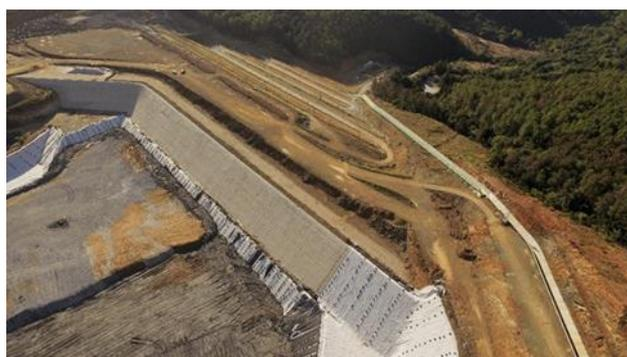
Figure 9. Downstream embankment construction.
