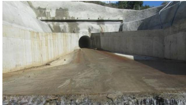
**Figure 3.** Diversion tunnel exit portal.
