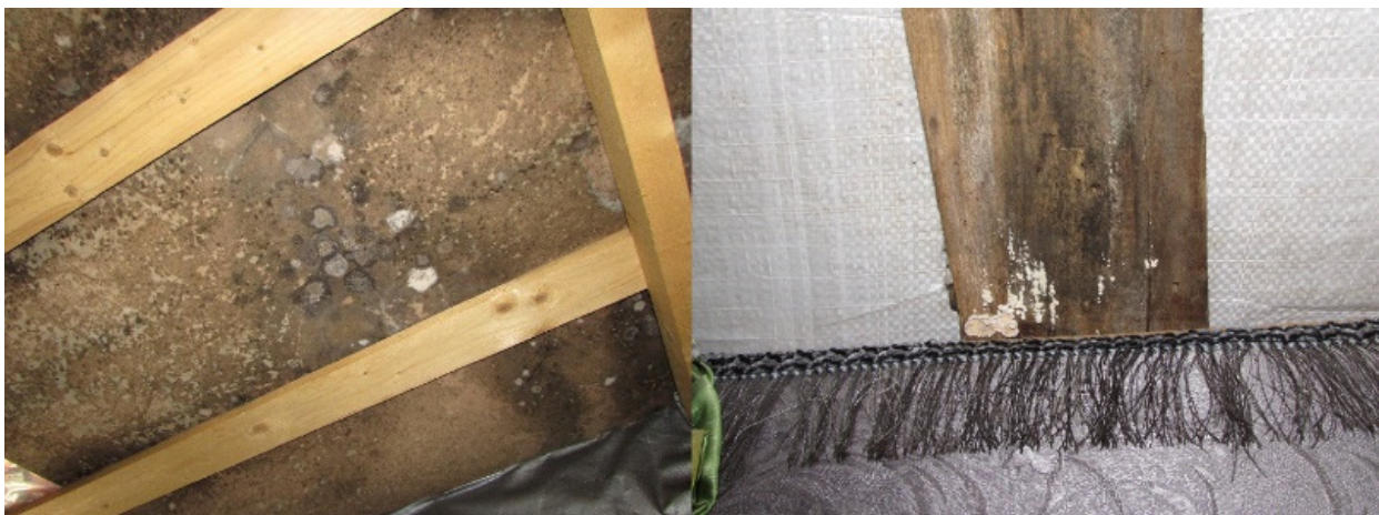
Figure 3. Example of mold growth on the ceiling ( left ) and wall ( right ) wood panels inside informal settlements.
