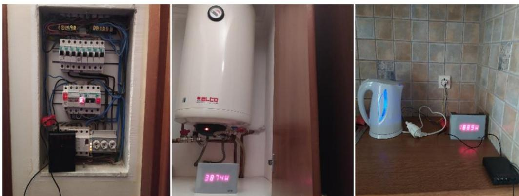
**Figure 3.** Smart meter configuration for data sampling.
