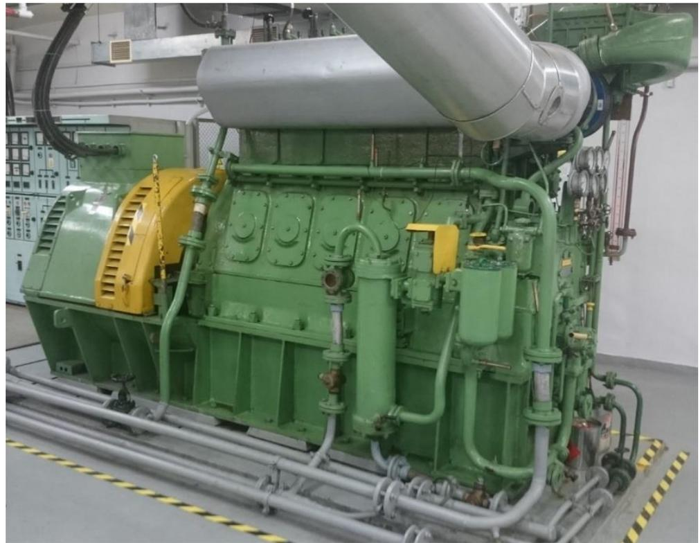
**Figure 1.** Sulzer 5 BAH 22 engine and associated circulating lubrication system.
