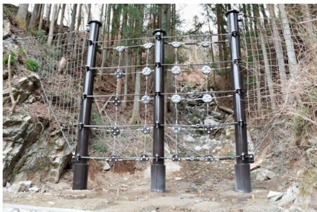
**Figure 1.** Example of secondary manufactured products (permeable debris flow barrier) and measures to prevent sediment runoff from the side (with wire mesh) in small-scale streams [21].
