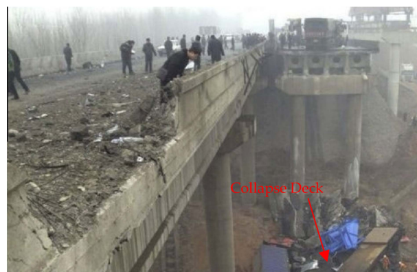
Figure 5. Collapse of the Yichang Bridge, Sanmenxia, Henan, China (reproduced with permission from Wang, W.; Liu, R.; Wu, B., Engineering Failure Analysis ; published by Elsevier, 2018) [85].
