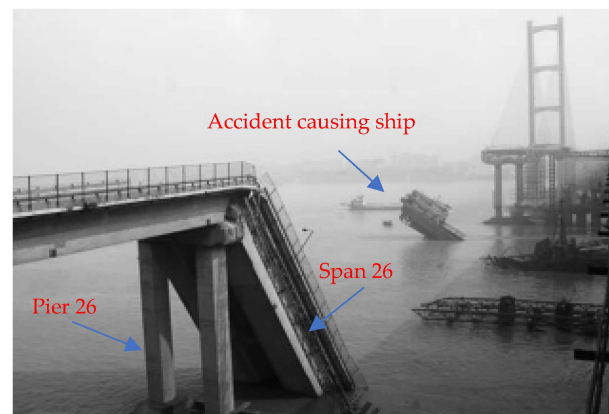
Figure 6. Collapse of Jiujiang Bridge, Foshan, Guangdong, China (reproduced with permission from Lu, Y.E.; Zhang, L.M., Ocean Engineering ; published by Elsevier, 2013) [89].
