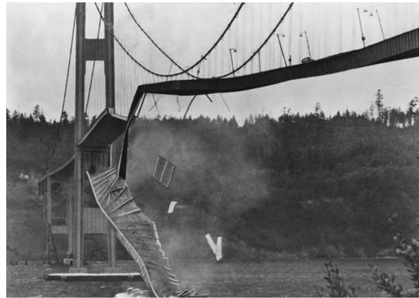
Figure 1. Collapse of the Old Tacoma Narrows Bridge, Seattle, WA, USA (reproduced with permission from Olson D. and Hook J., The Physics Teacher ; published by AIP Publishing, 2015) [2].
