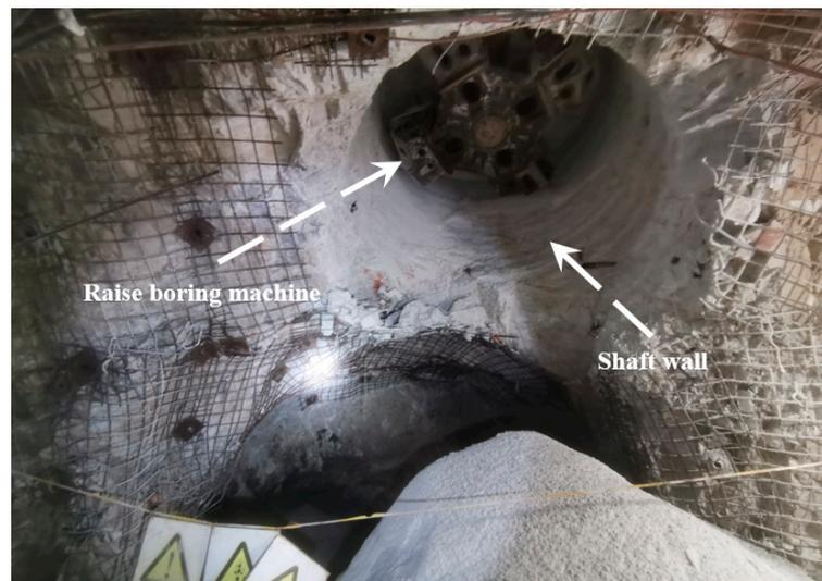
**Figure 3.** An ore pass drilled using a raise-boring machine.
