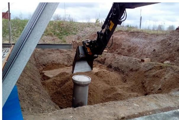
**Figure 3.** Construction of the test pit and filling with the material to be tested.
