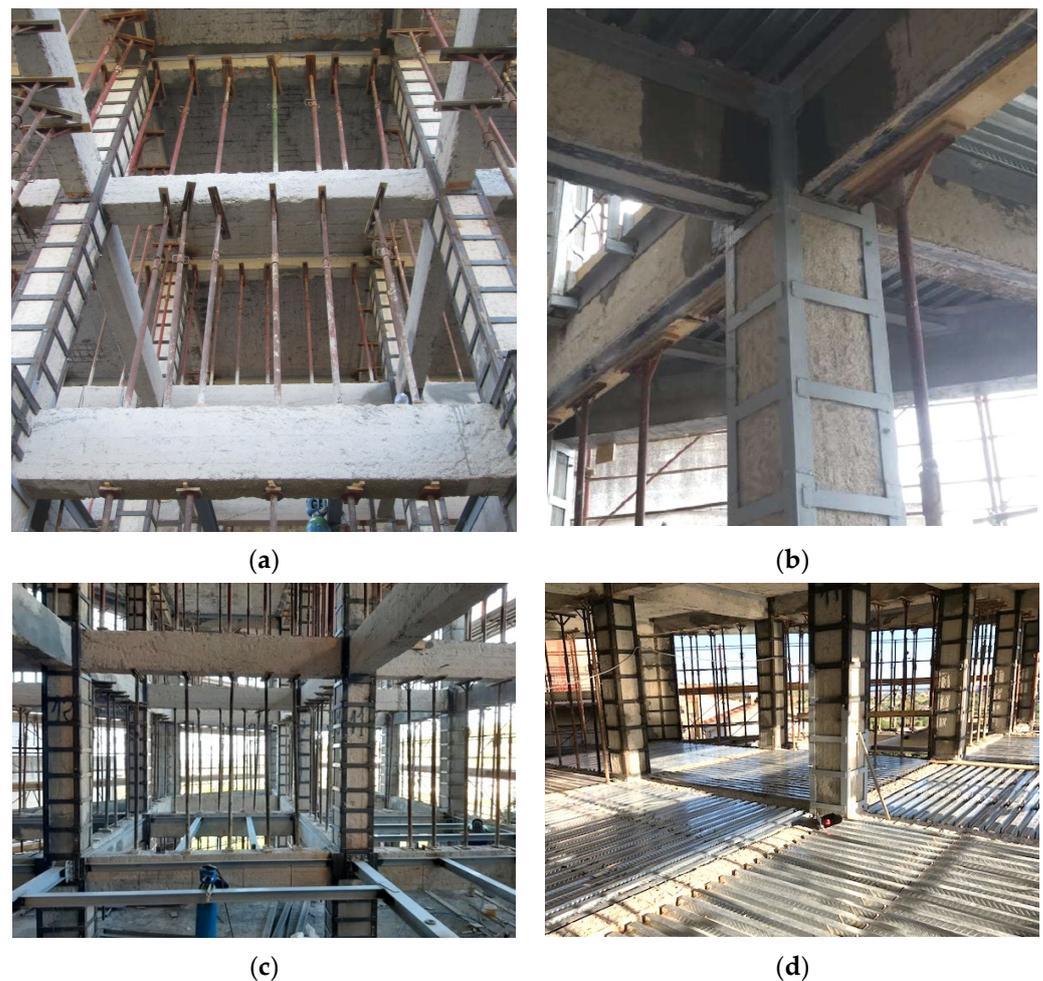
**Figure 9.** Views of retrofit interventions with steel jacketing and exoskeleton. (a) Shoring of beams during assembling of angles and battens; (b) Retrofitted columns; (c) Completion of columns retrofitting and new steel floor assembling; (d) Preparing in situ casting of floor slab.
