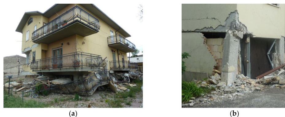
Figure 2. L'Aquila, Italy—2009: (a) damages on RC structure in L'Aquila; (b) node damage of reinforced concrete elements.
