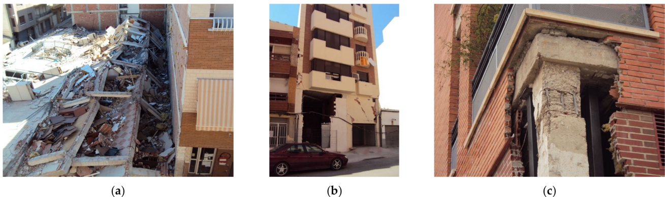
Figure 3. Lorca, Spain—2011: (a) building collapse after the earthquake; (b) building with a soft-storey mechanism; (c) column failure due to inadequate detailing of the transverse reinforcement.
