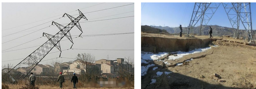
Figure 1. Transmission tower damaged by foundation settlement.
