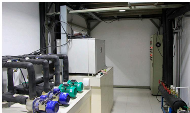
**Figure 10.** Real picture of the machine room of variable flow air conditioning water system.
