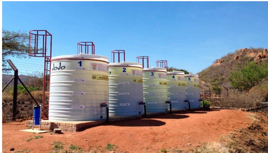
**Figure 3.** Photobioreactors at the Motetema wastewater treatment pond system implemented during Phase 2 [30].
