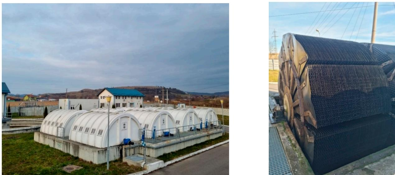
**Figure 2.** The RBCs of Agnita: the modules (left), and discs (right).
