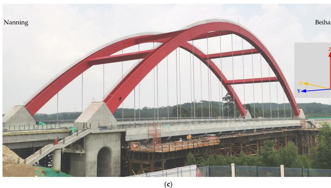
**Figure 3.** The layout of arch-rib-alignment-monitoring points: (a) schematic diagram of general layout of measuring points; (b) schematic diagram of side layout of measuring points; (c) schematic diagram of X, Y, and Z directions.
