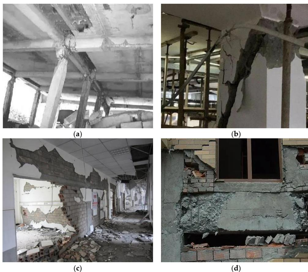
**Figure 2.** Damage patterns in RC structural members after seismic hazards. (a) Damage to joint elements; (b) Damage to column elements; (c) Damage to wall elements; (d) Damage to beam elements.
