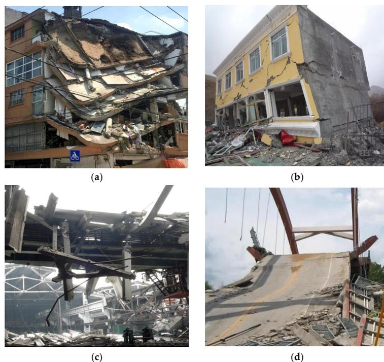
**Figure 1.** Damage phenomena of RC structures under real earthquake load. (a) Damage to residential building; (b) Damage to public building; (c) Damage to industrial building; (d) Damage to bridge.
