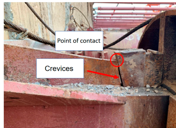
Figure 7. Local contact of steel wedge.
