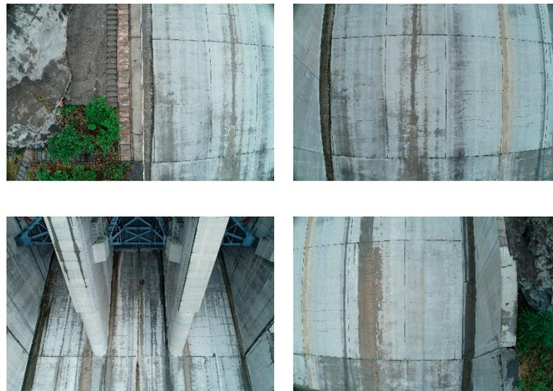
Figure 10. Crack samples of the spillway.
