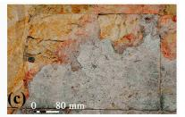
**Figure 1.** Degradation forms of the Calcari di Cagliari limestones: (a) alveolization of the Pietra Cantone; (b) loss of material and pulverization in a wall built with Tramezzario ashlars; (c) detachment and oxidation in a Pietra Forte ashlar.
