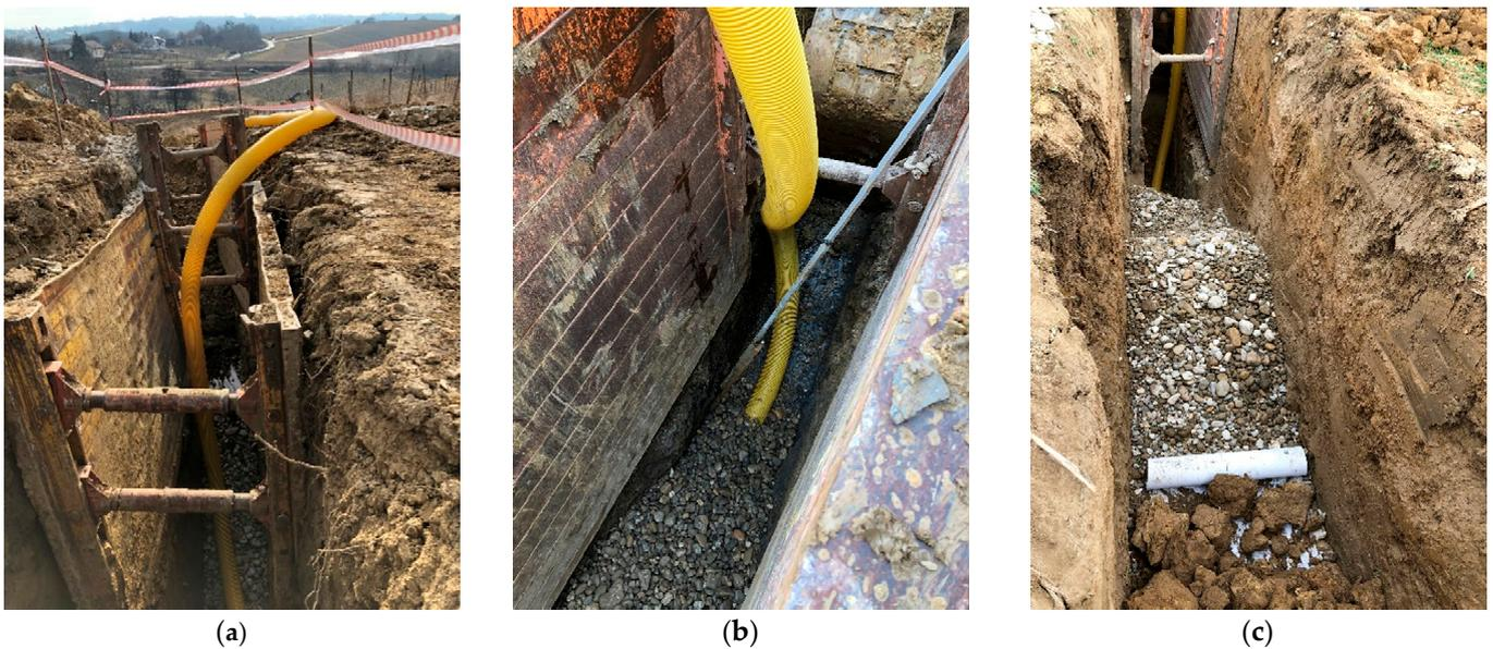
Figure 20. Building of the deep drain on the Orehovčak landslide: (a) excavation protection; (b) installation of perforated drainage pipe; (c) backfilling drain with drainage material.
