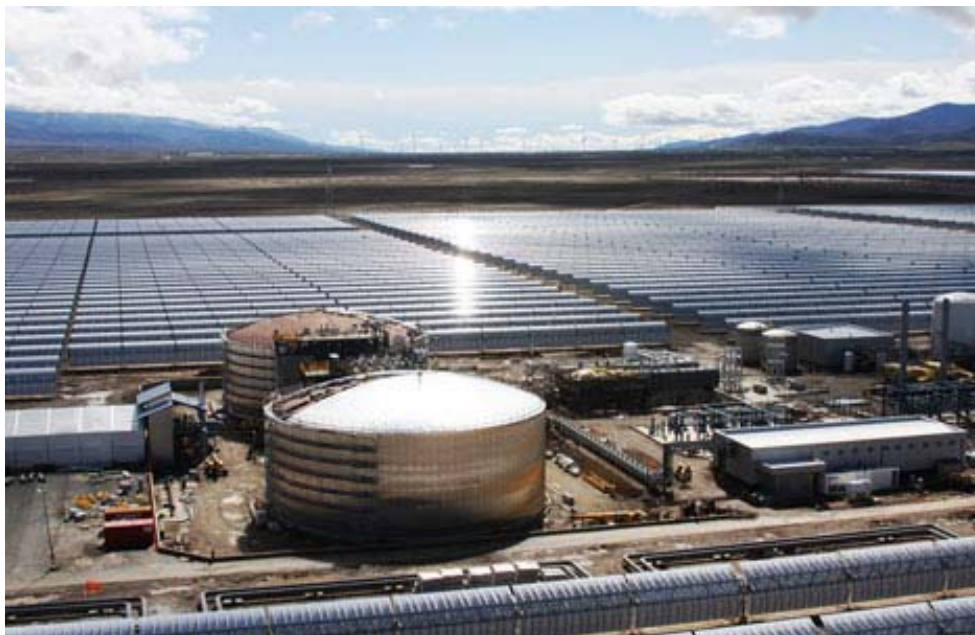
Figure 12. 50 MW Solar power plant Andasol 1 with solar thermal energy storage system [27], photo with permission from Solar Millennium.
