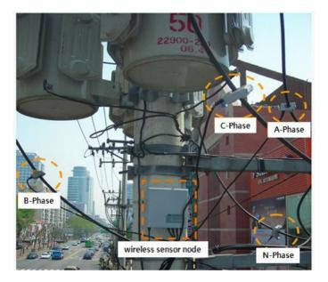
Figure 3. Wireless sensor node design on a pole transformer.
