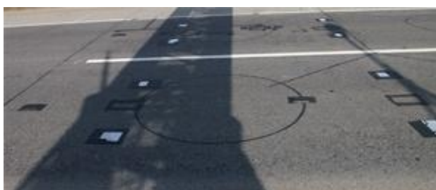
(b) Taped T-Sensor nodes and reflectors for the laser-based reference instrument on the pavement.
