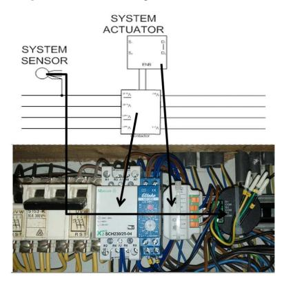
Figure 7. Kitchen stove coupled sensor/actuator device.
