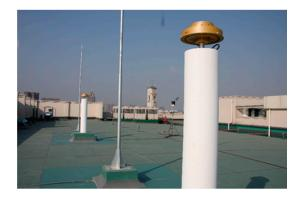
Figure 3. GNSS reference stations in UNNC.
