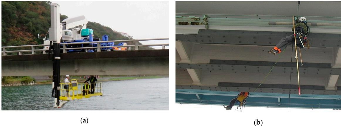
**Figure 1.** Example of inspection using a high-location work vehicle (a) and rope access (b).
