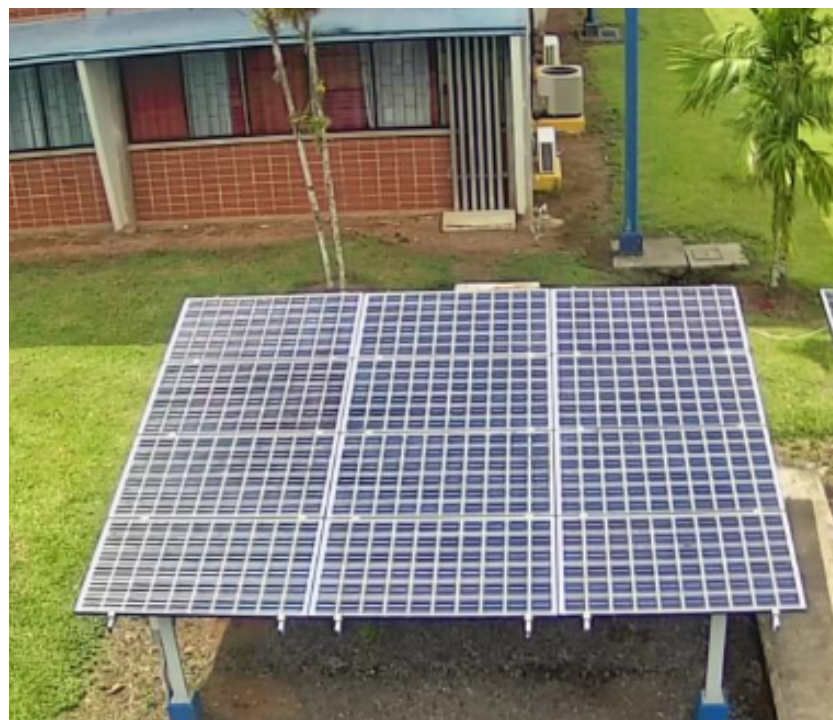
Figure 1. Polycrystalline 3.36 kW PV array used for this study.
